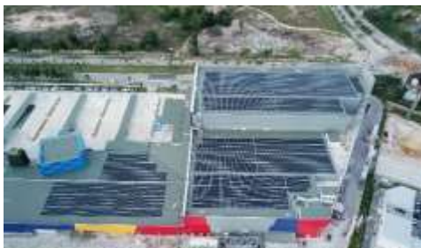
Sustainable Energy Services
