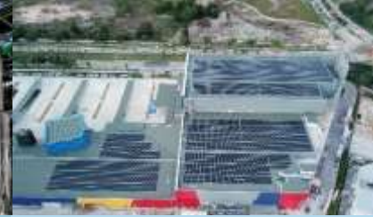
Sustainable Energy Services
